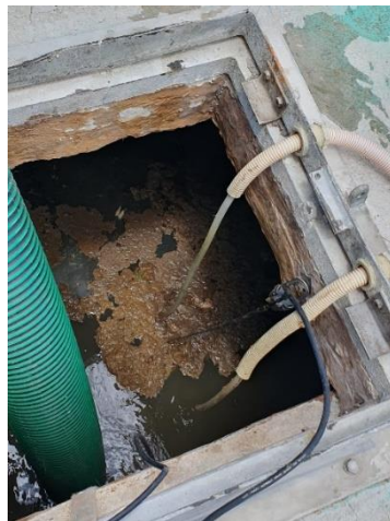
Figure 1. Images of Fat, Oil, Grease (FOG) discharges into sewer system Bubali area, taken June 2023. (Left) (brown) FOG at pumping station. (Right) Wastewater overflow onto public domains.
